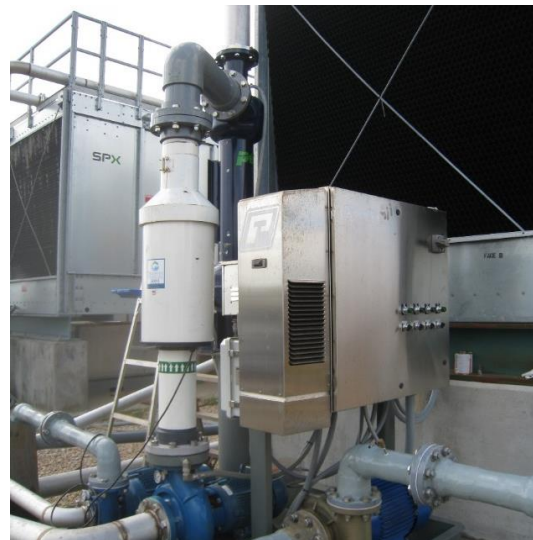
Electronic Centrifugal Filter
